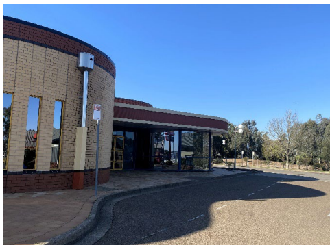
Image: Western elevation of the ACMHF
