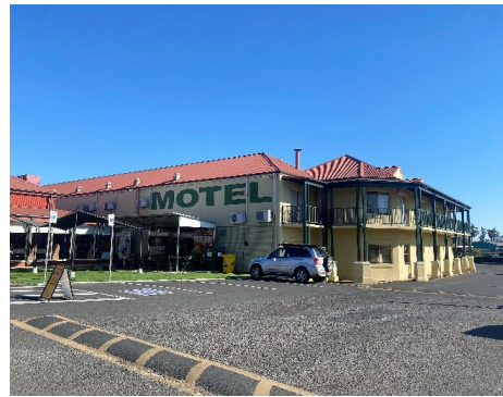
Image 4: View Northwest to the motel adjacent the Visitor Information Centre
