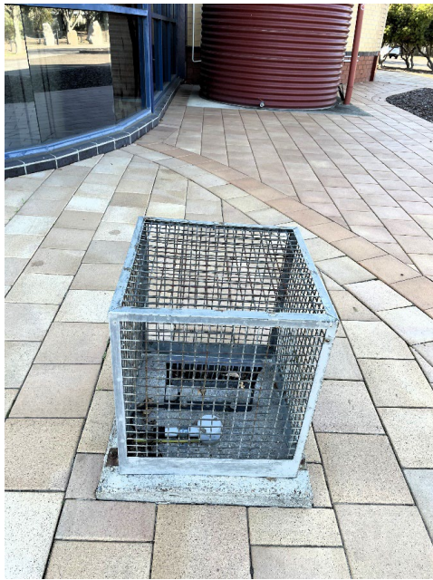
Image: ACMHF external paving and lighting detail
