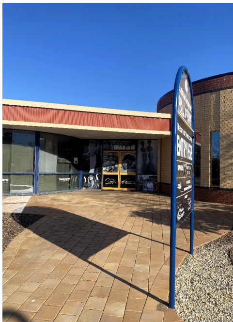
Image: ACMHF eastern façade disused museum entry and directional signage.
