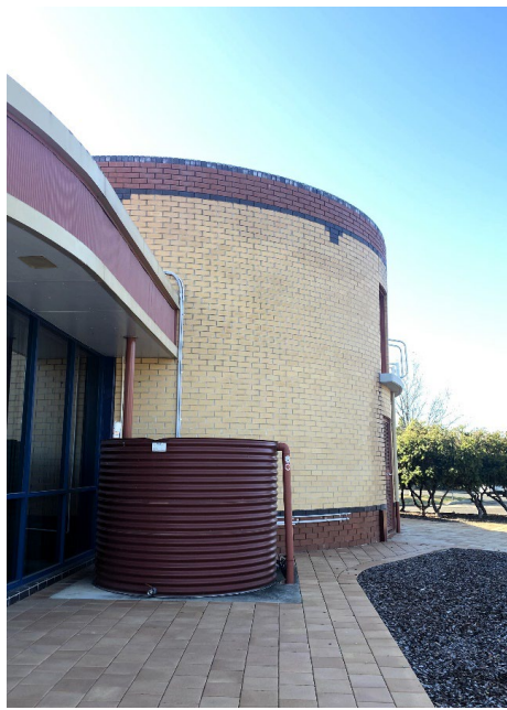
Image: ACMHF façade with rainwater tank
