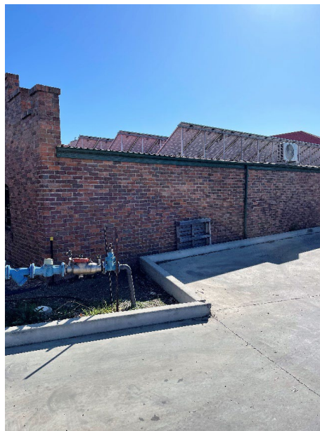
Image 12: Visitor Information Centre Southern Façade from KFC carpark with PVs on the roof.
