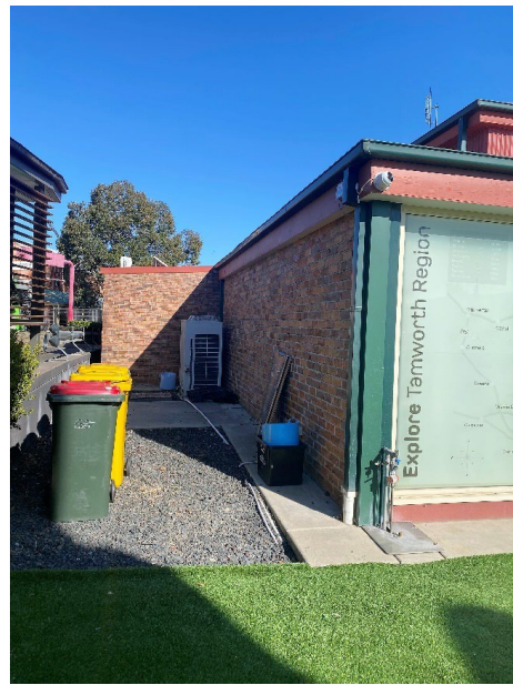
Image 6: View of the Southern façade of the Visitor information Centre
