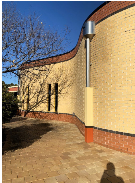
Image: ACMHF eastern façade detail with stainless steel downpipe and paving
