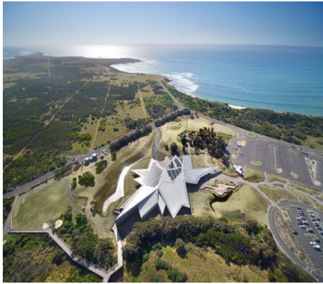
Image: Aerial View of the facility
