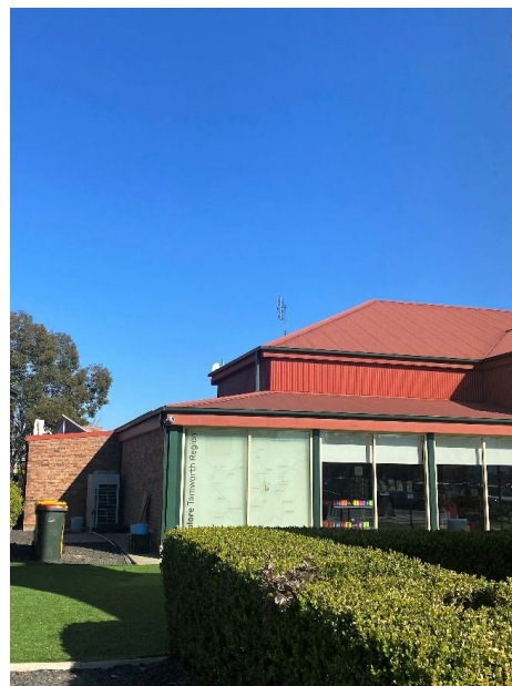
Image 10: Visitor Information Centre glazed Eastern Façade
